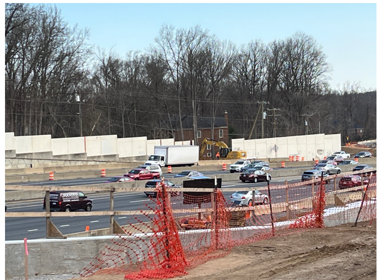
Viewed from across the Beltway, crews have removed a two-panel section of noise wall along Live Oak Drive (photo taken March 12).
