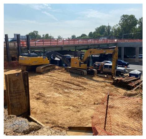
Steel piles will be driven into the earth at this location, which is adjacent to the existing Georgetown Pike Bridge and between the onramp to northbound I-495 and the Beltway.
